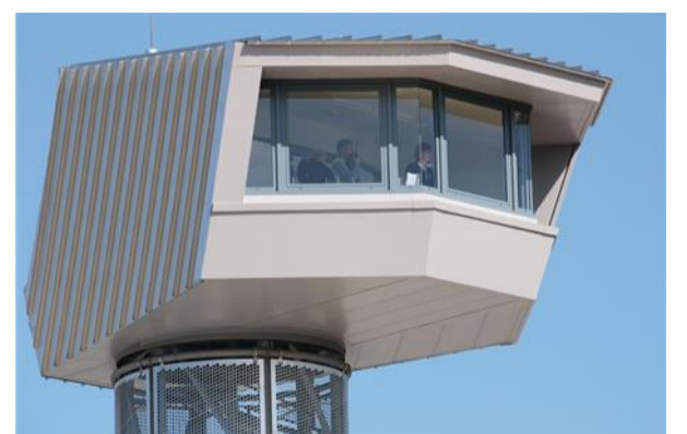
The control tower
