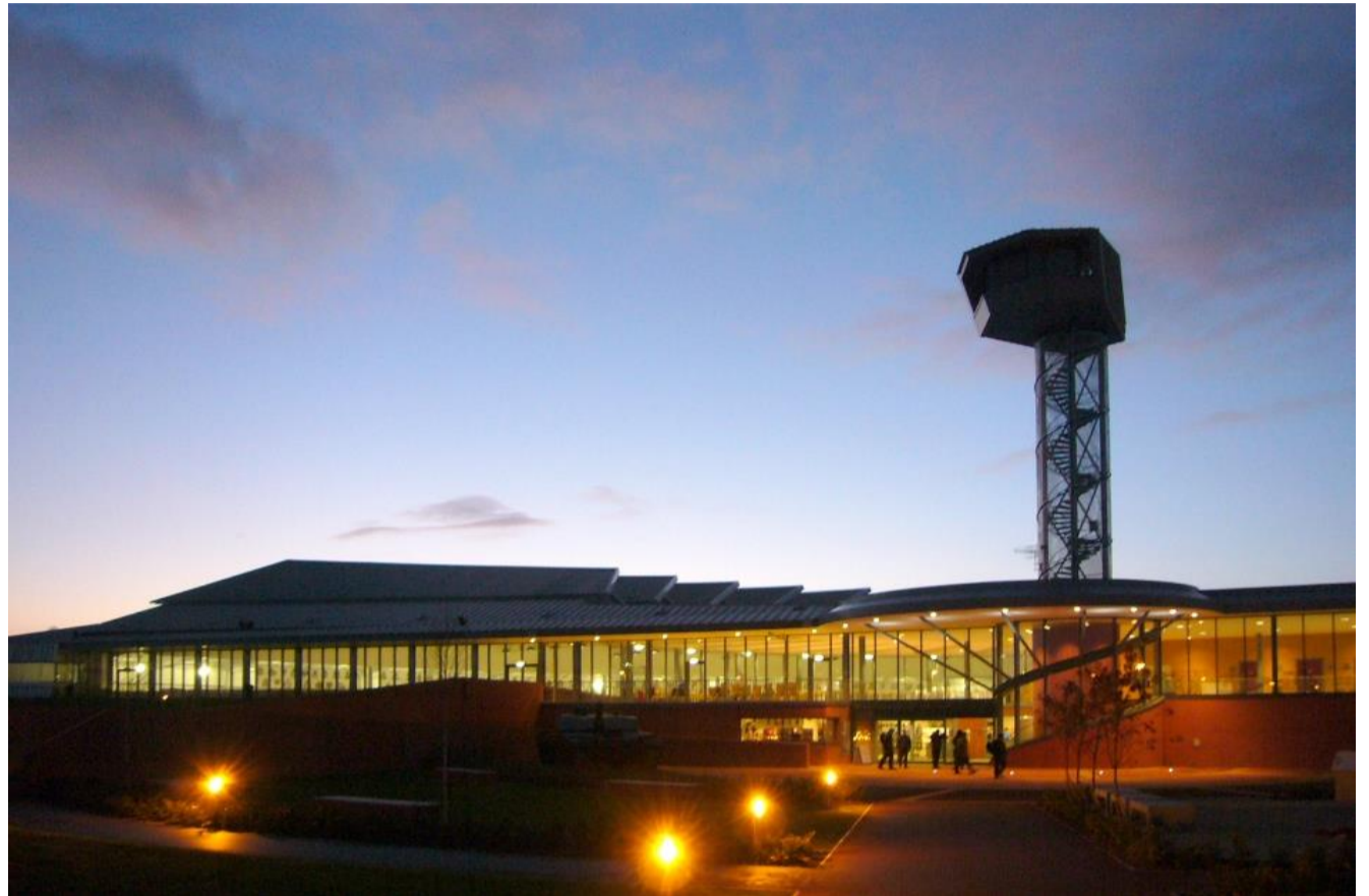
The new entrance and display hall. The tower is used to orientate visitors on the 12-hectare site and to control the 'tank in action' events in the arena below
